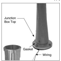
**1.** Remove top of junction box and disconnect wiring splices.
